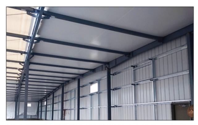
AutoCeil System pulls sheet in minutes and covers ceiling and both side walls. System is tensioned, secured and ready for insulation.
