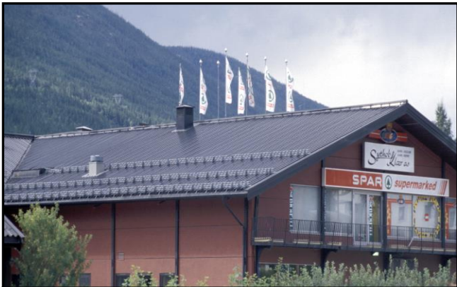
Figure 9: This project in Norway demonstrates appropriate placement of multiple rows, concentrated in the lower half of the roof
