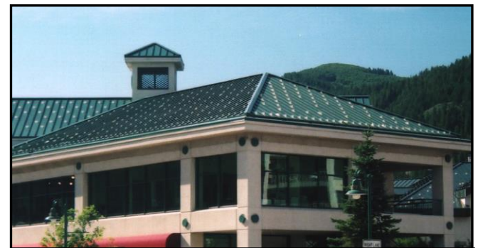
Figure 8B: “Cleat” type snowguard system
